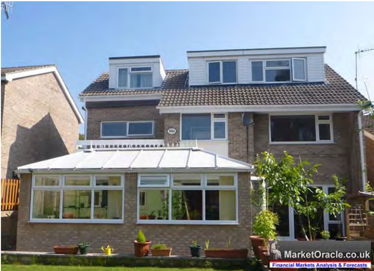
After loft dormer conversion:
